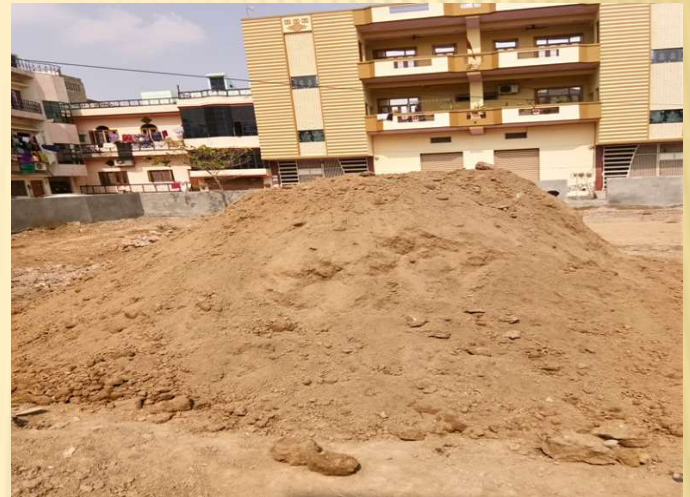
Cleaning and filling work at site
