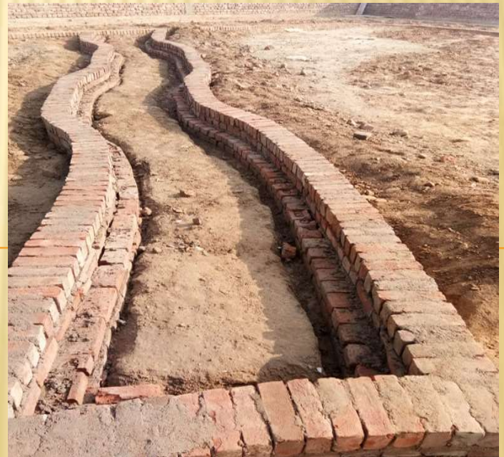
Fountain work progress in park
